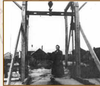
Construction of bridge in village
