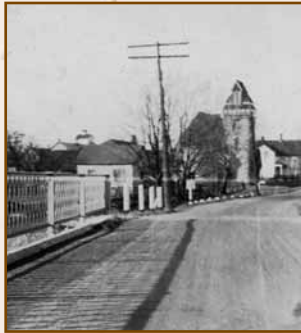
First of 3 Bridges located on planked road (Hwy 43) in Port Elmsley
